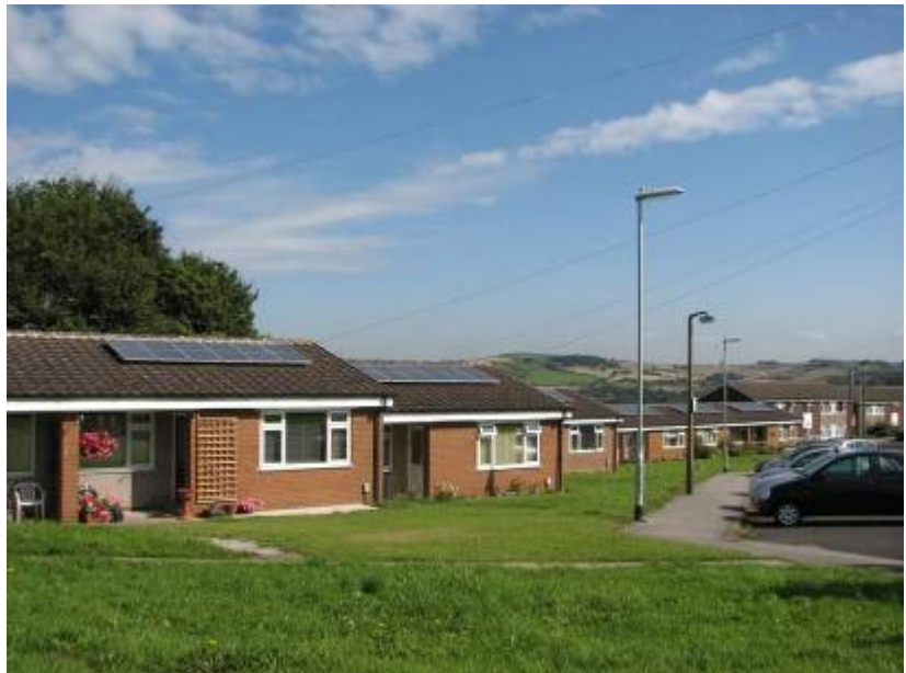
PV on housing association properties in Fernside
